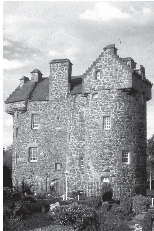
Claypotts, Dundee (author). The clumsiness with which the original caps of the towers have been replaced by the rectangular studies c.1588 implies that a very public point was being made.
