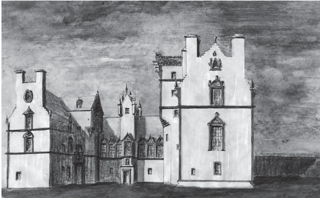
Wrichtishousis, Edinburgh, villa of the Napier family, demolished 1800 (conjectural reconstruction by the author based upon drawings by Alexander Nasmyth and others). A gallery separates the family wing (left) from the public/ guest wing on the right.
